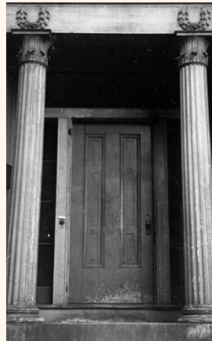
James Munroe Jr. house, 127 Mt. Auburn Street. Portico with fluted columns, Temple of the Winds capitals, and wreaths. D. Wetherell photo, ca. 1935.
