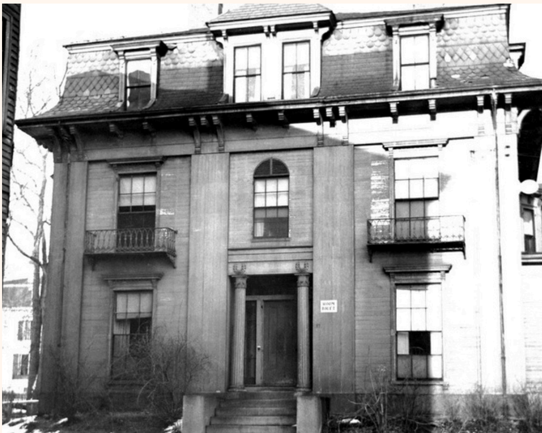
James Munroe Jr. house, 127 Mt. Auburn St. (1845, William Hovey, architect). The Mansard roof and brackets were added ca. 1868. The entrance columns with acanthus capitals were removed in the 1960s. Photo ca. 1950.
